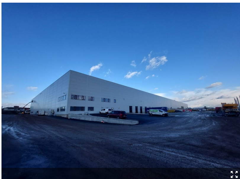
CTP-Park Vienna East
